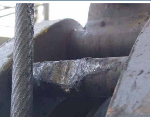
Picture 5: Contact between rope and crane construction points
